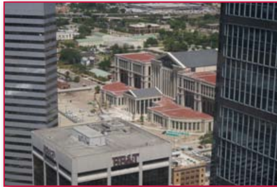
The nearly completed Duval County Courthouse taken from the River Club (The courthouse opened for business on June 18, 2012)
